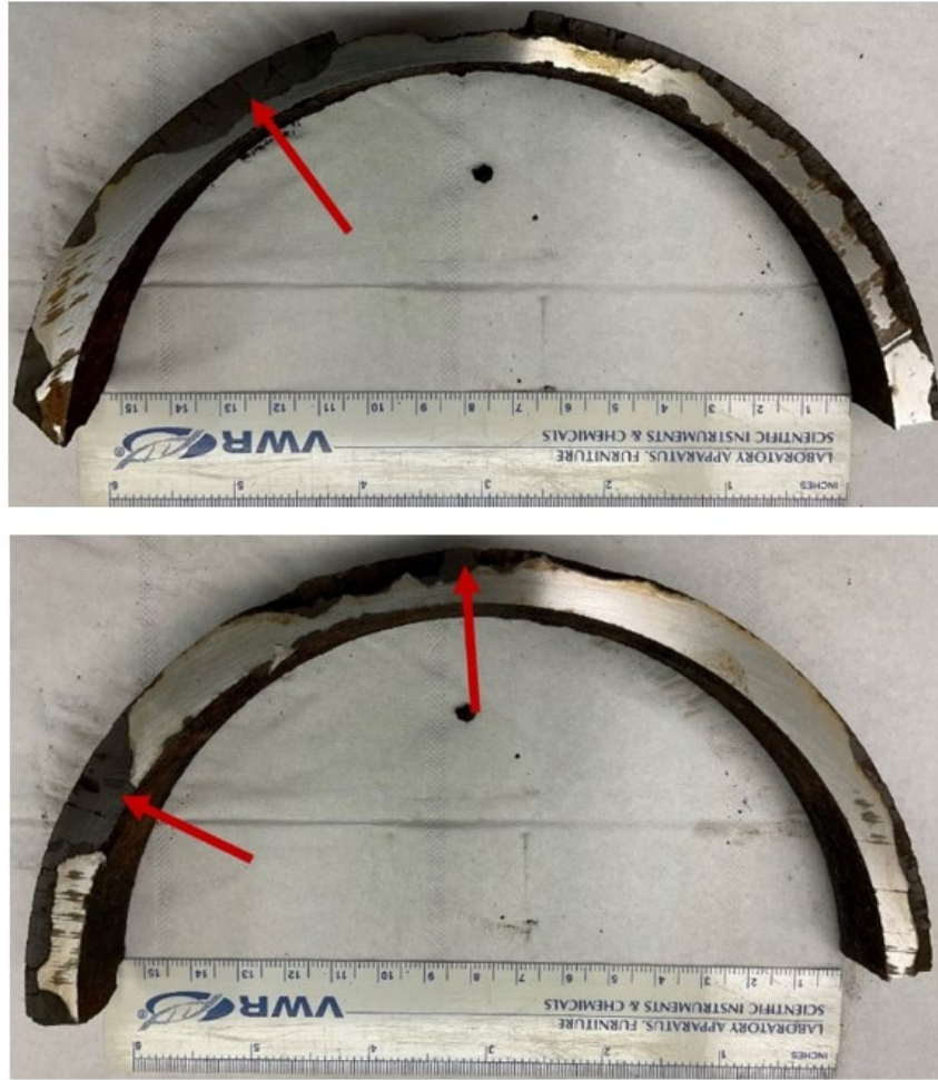
Figure 18. Photos of cross sections of the rings cut from the corroded cast iron pipe. Shiny areas are unaffected metal while the dark areas are the oxide corrosion product. Photos show areas of significant corrosion. In the bottom photo note the area of through-wall corrosion on the far left side.
